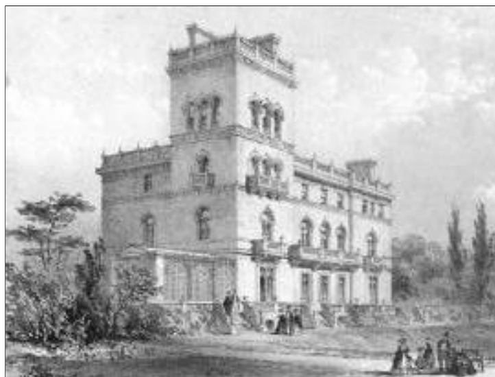
No. 8, which was used for the interrogation of spies during the Second World War, was in 1961 replaced by an apartment block.
